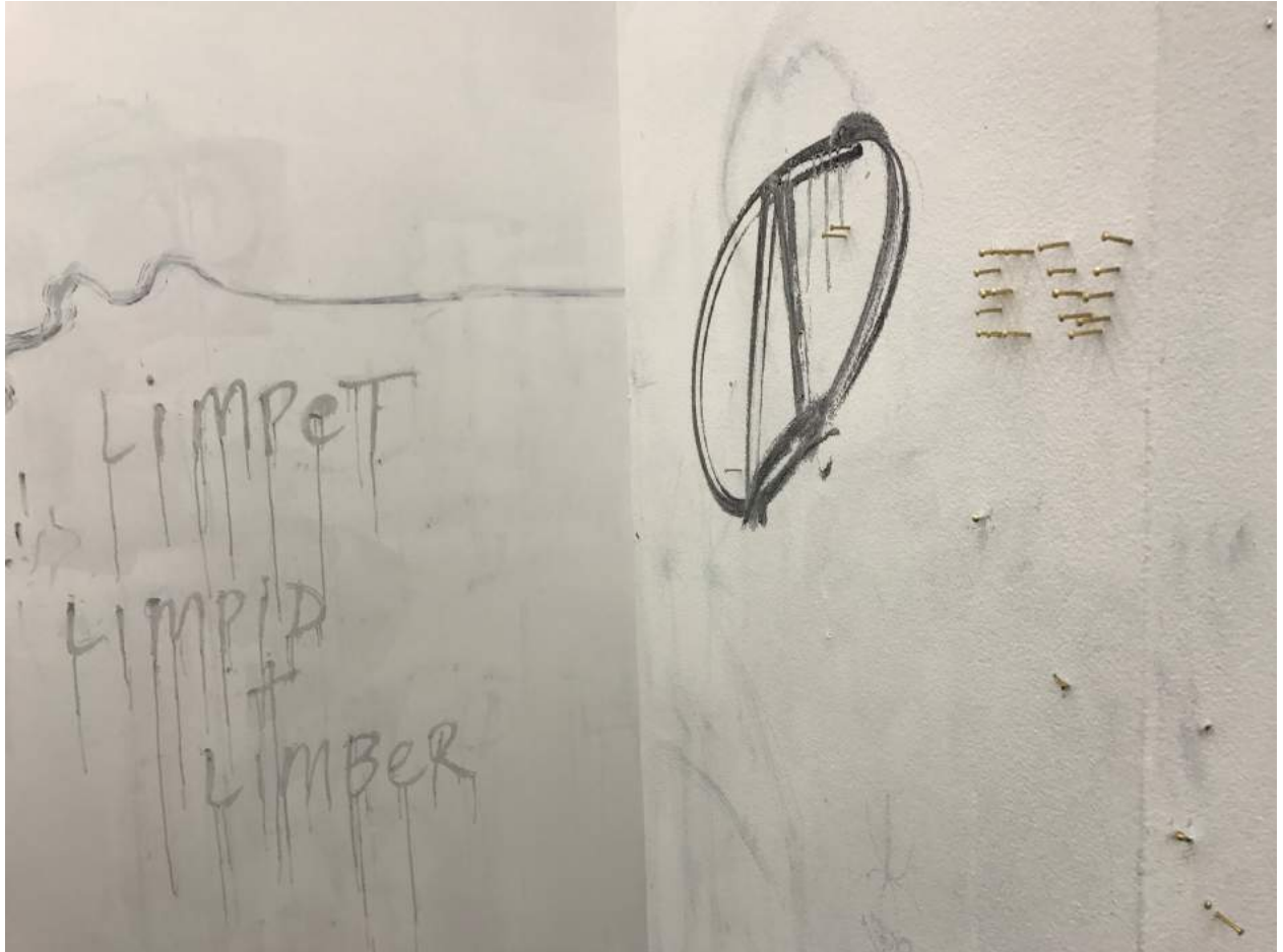
Detail: pillar and north wall, March 18, 2017
